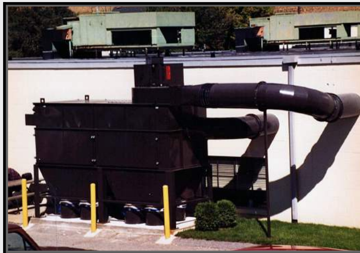
Above: Dust Collector Unit Outside Facility
