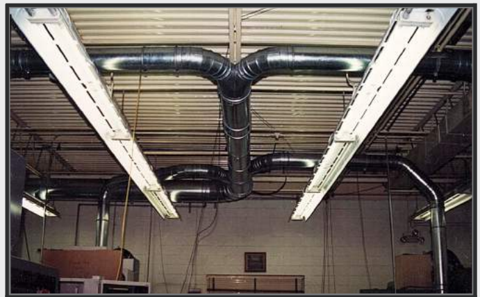
Above: Ducting installed in Key facility
