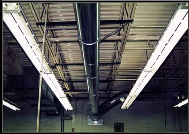
Above: Example of Straight Duct Work
