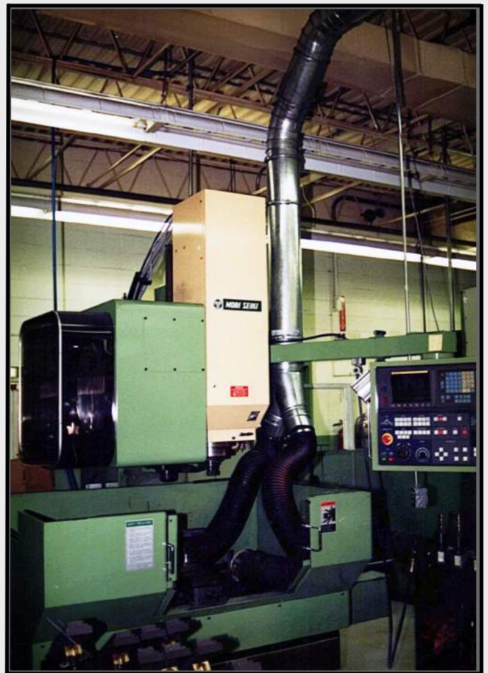
Above: Precise Ducting From the Work Area
